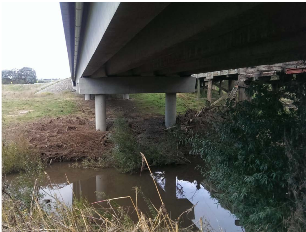
Photograph P9 - The current and former Gundaroo Bridge – March 2014
