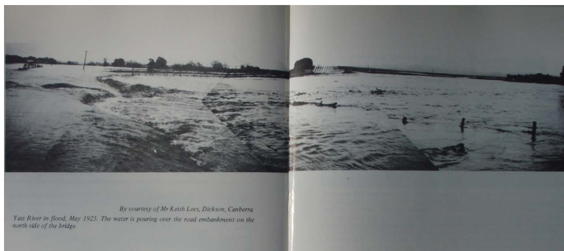
Photograph P7 - May 1925, floodwater across Sutton Road and beneath Gundaroo Bridge.
