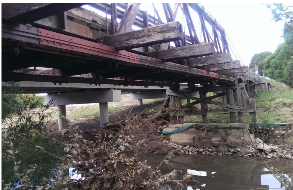
Photograph P10 - The current and former Gundaroo Bridge, looking east – 11 March 2014
