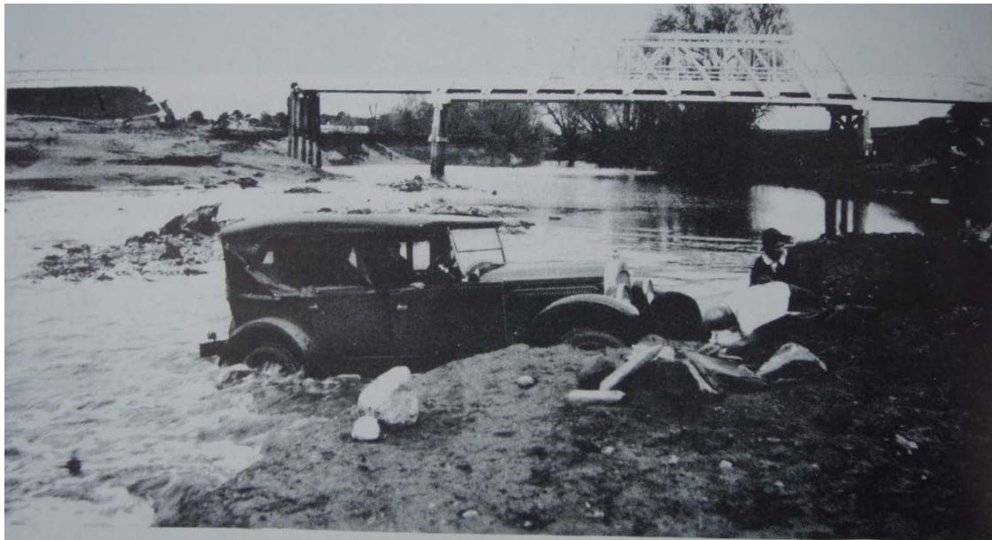
By courtesy of Mrs Frances Sibley, Queanbeyan. 25. Crossing the river after the flood. Part of the embankment was washed away by the flood.
