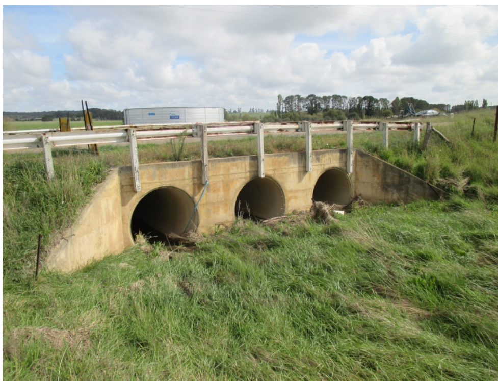
Photograph P1 – Upstream view of the 3 x 1.8m diameter pipe culvert conveying flow in Harrow Creek under Sutton Road.
